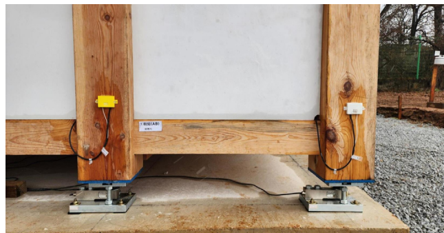
Fig. 12. Damage to the lower part of the column
